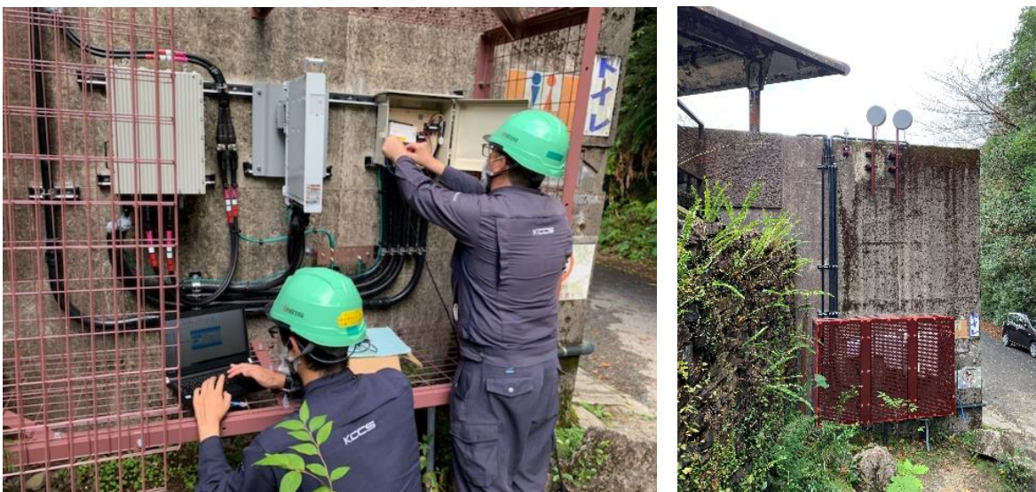
Fig. 12 Communication zone countermeasure work (left) Base station and small, circular antenna (right)
